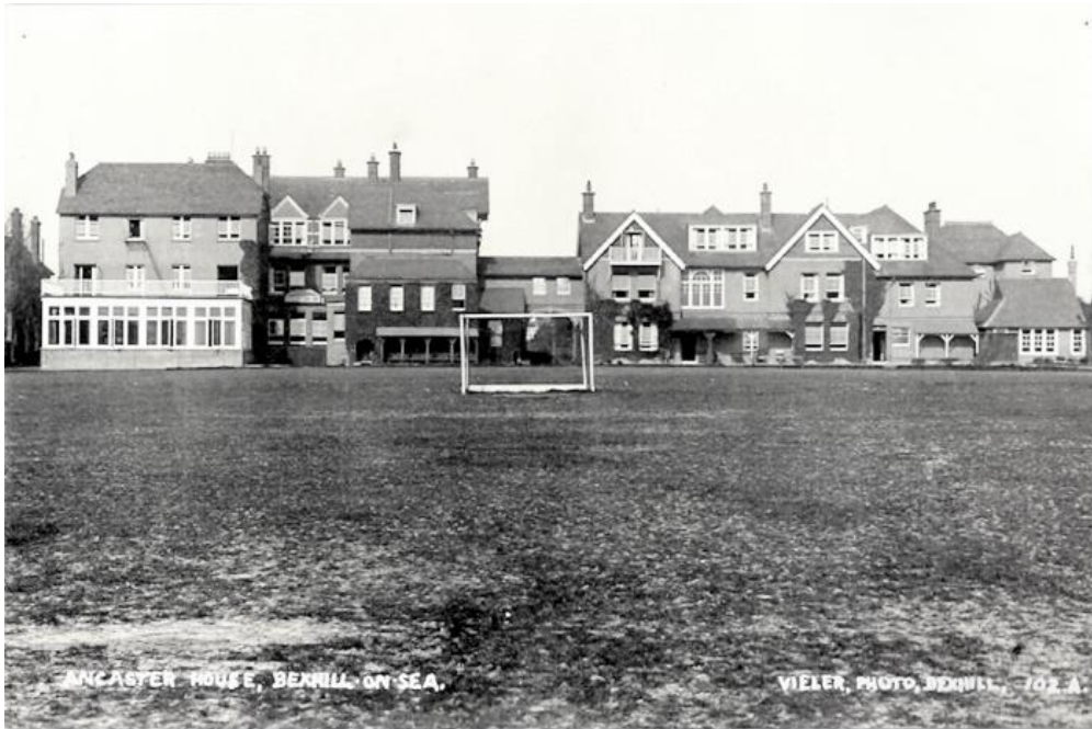
Ancaster House, Penland Road. (Rear view from playing fields)
