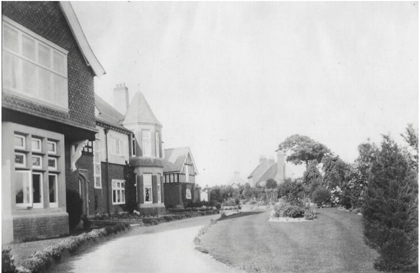
View of the drive and main entrance
