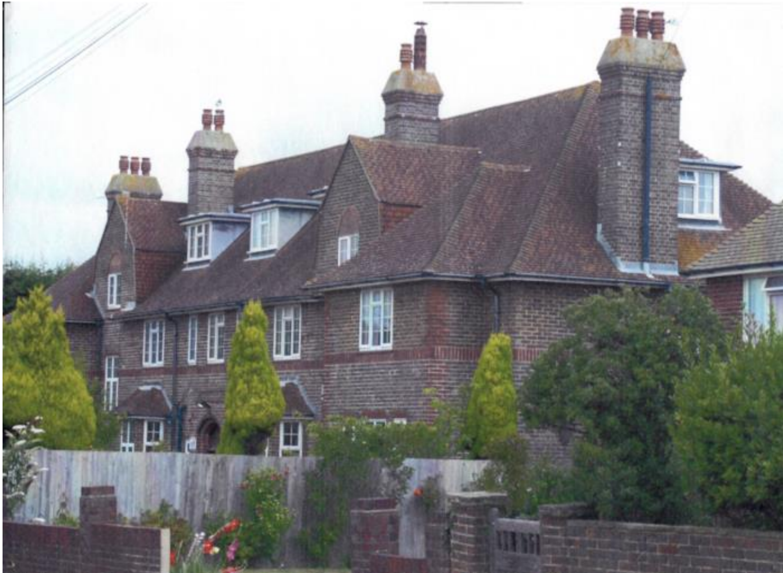
The outside of the building
