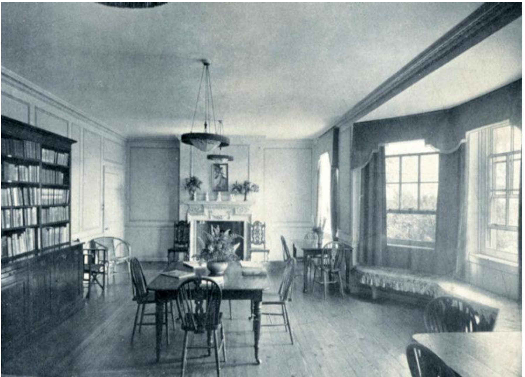
Below is a view of the girls "Common Room".
