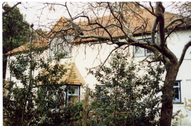
Two views of Whitehouse Farmhouse in Pembury Grove taken 1989
