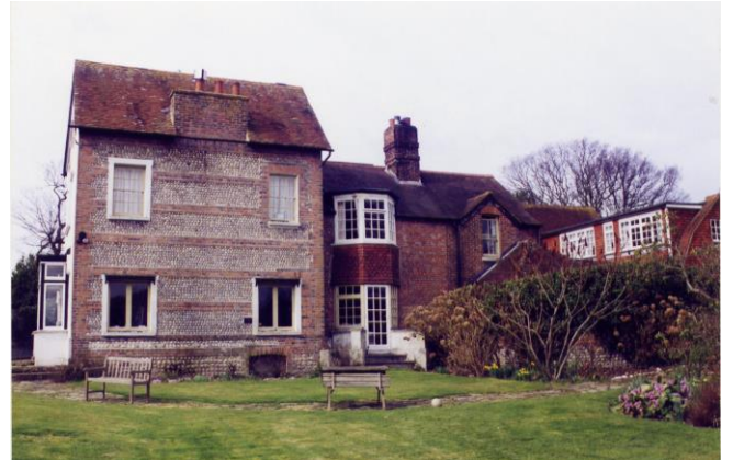
East side of house
